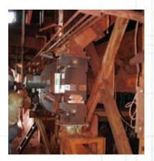
IRON ORE/TACONITE WINDBOXES (ANNULAR COOLER)
